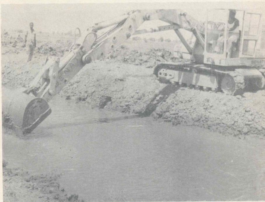
A modern dredger being used in the cleaning of an irrigation canal.
